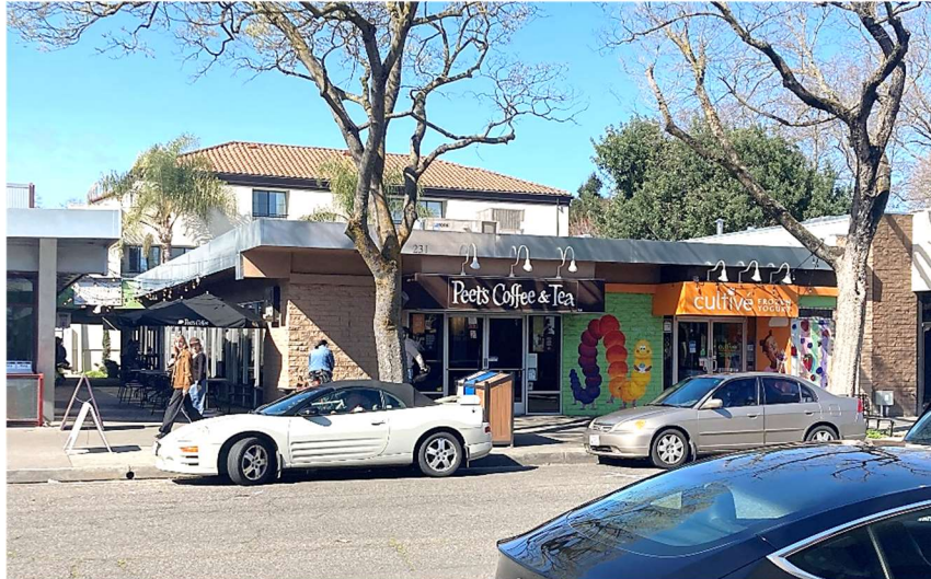
Primary (east) façade of 231 E Street, view facing northwest, ESA 2024.
