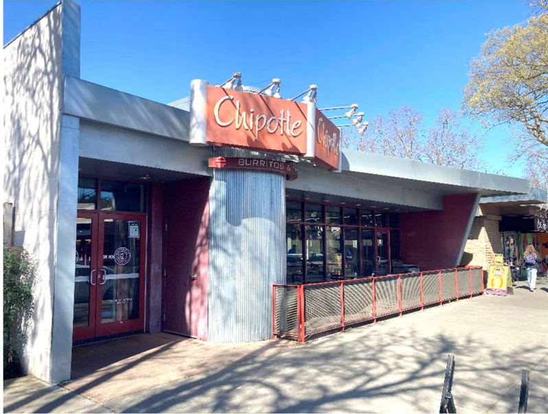
Primary (east) façade of 227 E Street, view facing northwest, ESA 2024.
